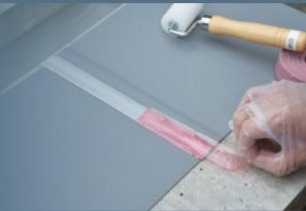
Cat-tape cures and bonds in 24 hours after application, and bonds strongly to both Catpad sheets and mortar foundation surfaces.
