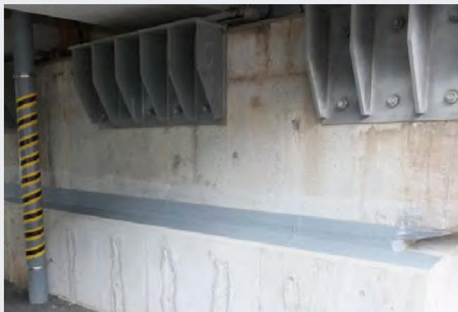
Waterproofing between the old column and the new concrete jacking prevents rainwater penetration into the joint of the concrete jacking. Long-term seismic resistance can be expected.
