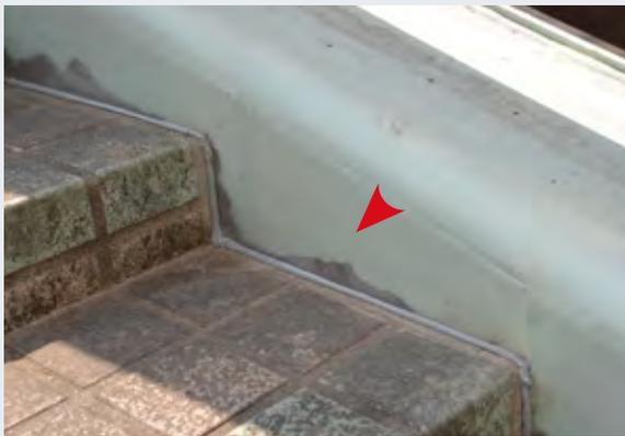
Catpad-Cloth was applied to the side wall of these steps. It prevented the formation of rust and prevented water from being trapped or stagnating from the flow of rainwater from the upper stages.
