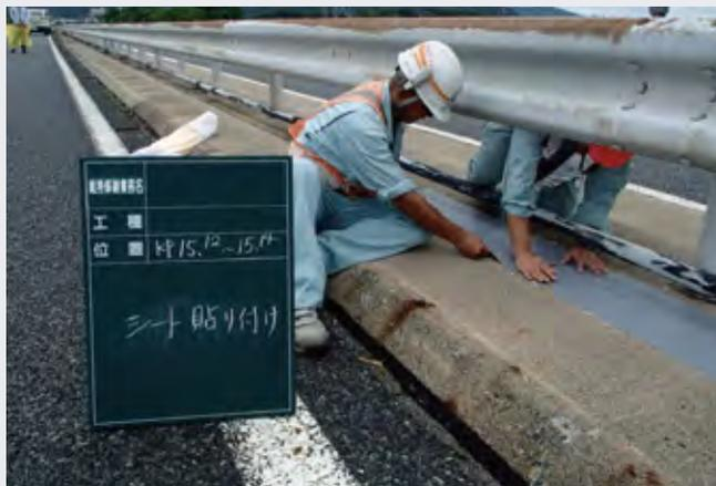
When applied to the median joints on intersecting roads, railways and bridges, Catpad shows superior weather resistance and durability compared to conventional polybutadiene resin, PVC and urethane waterproofing sheet.
