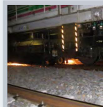
As part of ongoing maintenance rail grinding machines run to maintain the desired rail surface. Synthetic rubbers deteriorate due to sparks generated during grinding, but Catpad is hardly affected.
