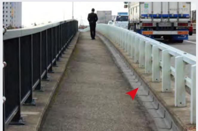
The system accommodates the differential movement of the carriageway and the pedestrian bridge maintaining a weatherproof seal and preventing water leaks.
