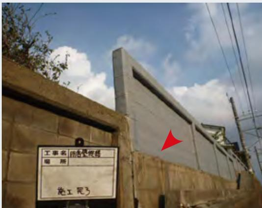
Applying Catpad all over the existing block wall surface, waterproofing, freeze-thaw damage prevention, and cleanliness were achieved.
