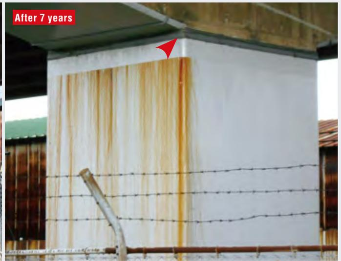
Catpad can be applied to both the coated steel and mortar without a primer. It will accommodate the combined movement of each substrate resulting from the difference in expansion coefficients of each material for long periods. Changes or an increase in corrosion can be checked by using Catpad Clear.
