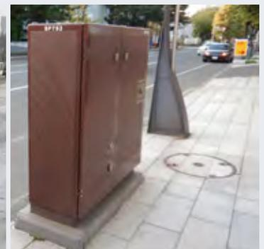
Prevents infiltration and freeze-thaw damage of street transformer base buried in snow for more than 3 months in winter.
