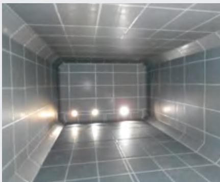
It successfully prevented deterioration and protected the water storage tank from potential damage caused by hot spring water.
