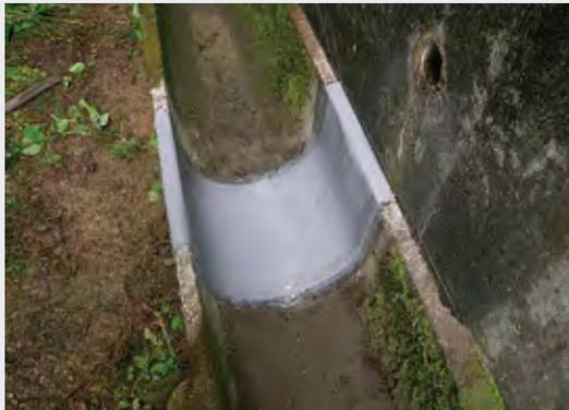
When compared to conventional mortar repairs, Catpad requires no mixing and is easy to apply without the need for specialist training. Once installed, it has a minimal curing time and can accommodate joint movement.
