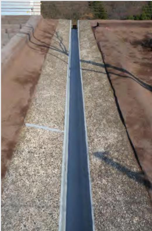
When normally replacing or repairing a U-ditch, heavy equipment such as a crane is required. This is no longer the case when the repairs are carried out using Catpad.
