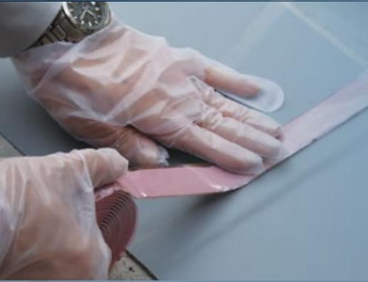
Cat-tape cures and bonds in 24 hours after application, and bonds strongly to both Catpad sheets and mortar foundation surfaces.
