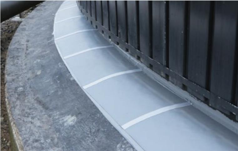
**Catpad, Catpad-cloth and Cat-tape used to protect metal cover against corrosion.**
