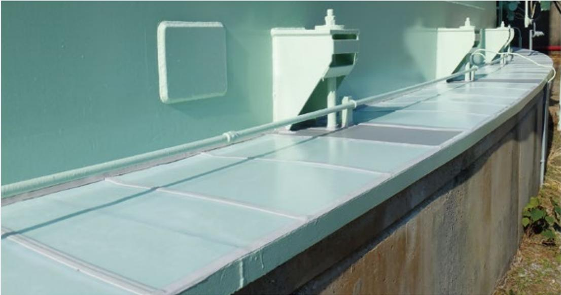
**Installation in which Catpad partly covers the wall of the foundation for a small tank.**
