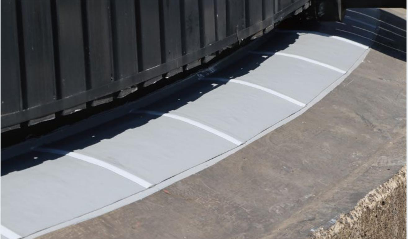
Shin-Etsu Silicone S COAT-57 has been used to eliminate low spots.
